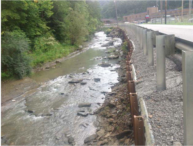
Railroad Rail Retaining Wall near school
